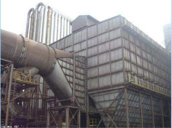
• Drop Out Box, Water-Cooled Duct, Fixed Duct
